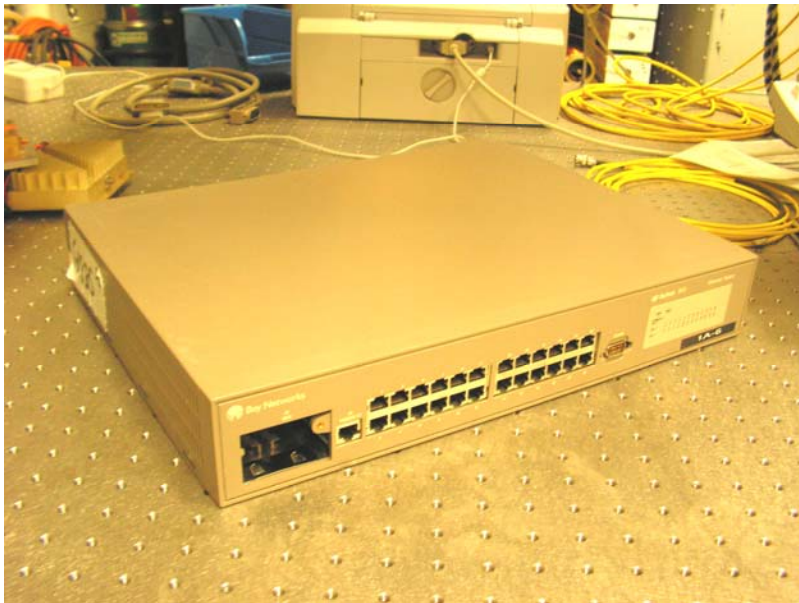
View of the assembled LAN switch
